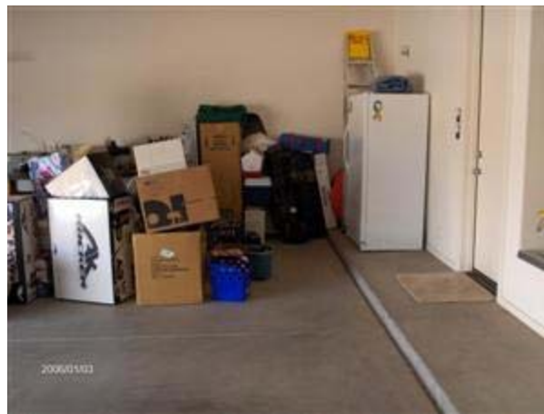
4.2 FLOOR SLAB Picture 1
