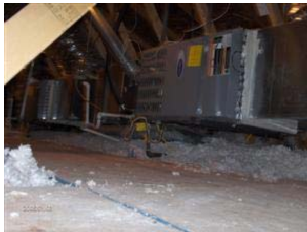
5.0 ROOF FRAMING Picture 1
