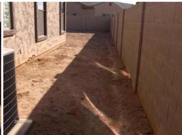
3.7 SITE GRADING Picture 2
