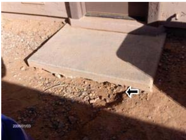
3.7 SITE GRADING Picture 1
